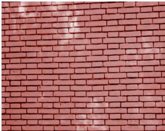
(a) Brick wall
